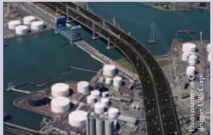
The proposed new Pearl Harbor Memorial Bridge, better known as the Q Bridge, is a $300 million project.
